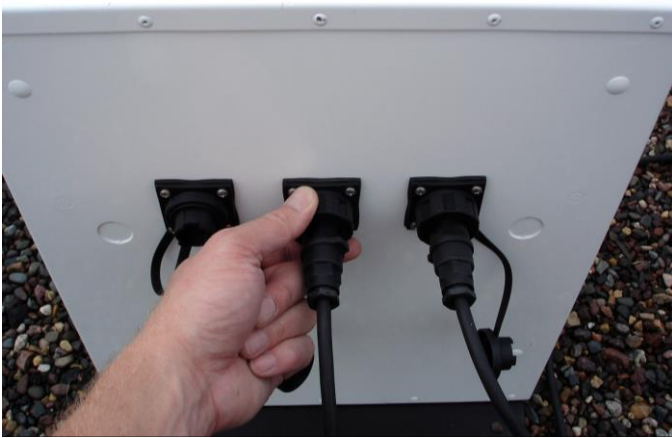
Figure 48: Connect Solar Cells to Battery Enclosure Box
